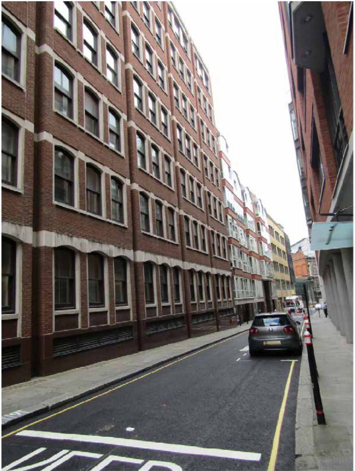
CASE No. 16/00215/FULMAJ Hosier lane, facing west
